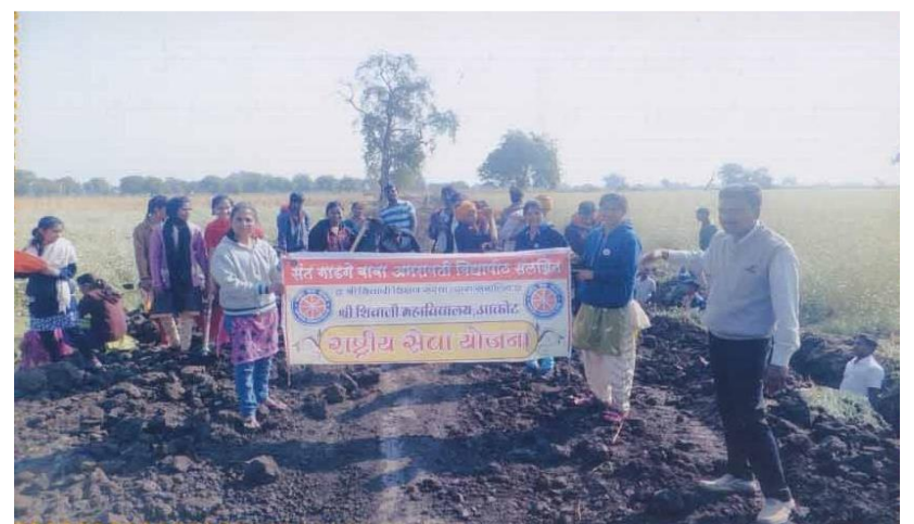
CONSTRUCTION FRAM LINK ROAD
