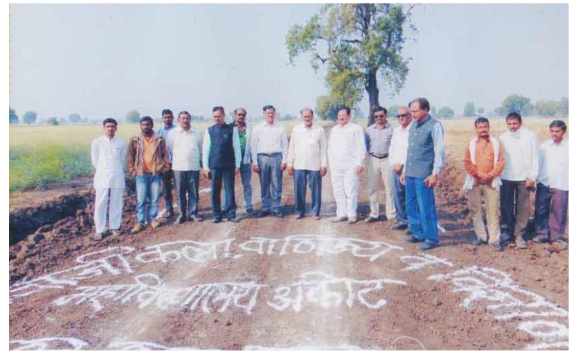
CONSTRUCTION OF FARM LINK ROAD
